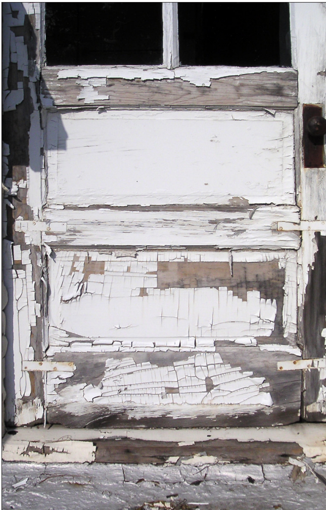
The paint at this door has alligatorated, with severe cracking visible. Paint loss has exposed bare wood. Both conditions allow storm water to come into direct contact with the wood surface, potentially leading to moisture deterioration. In this case, removal of all paint layers and proper door repair are recommended prior to repainting.
